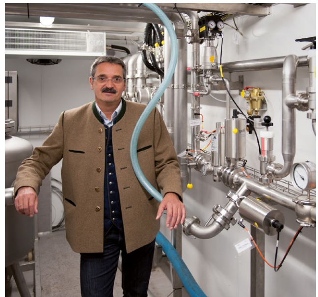
Fig. 1 Uwe Daebel, Department Head for Filling and Packaging Technology at Paulaner, was keen on the idea of maintaining a constant pressure and was impressed by the precision with which the hygienic right-angle valve with a 8049 digital positioner was able to maintain pressure.
